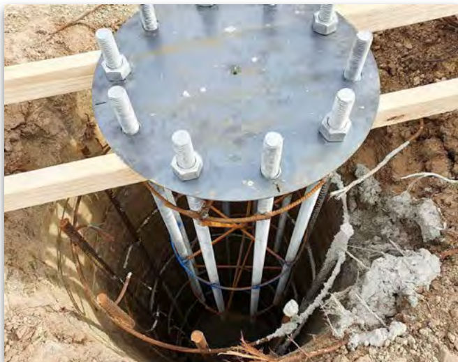
34 holes were dug, 6m deep and reinforced
