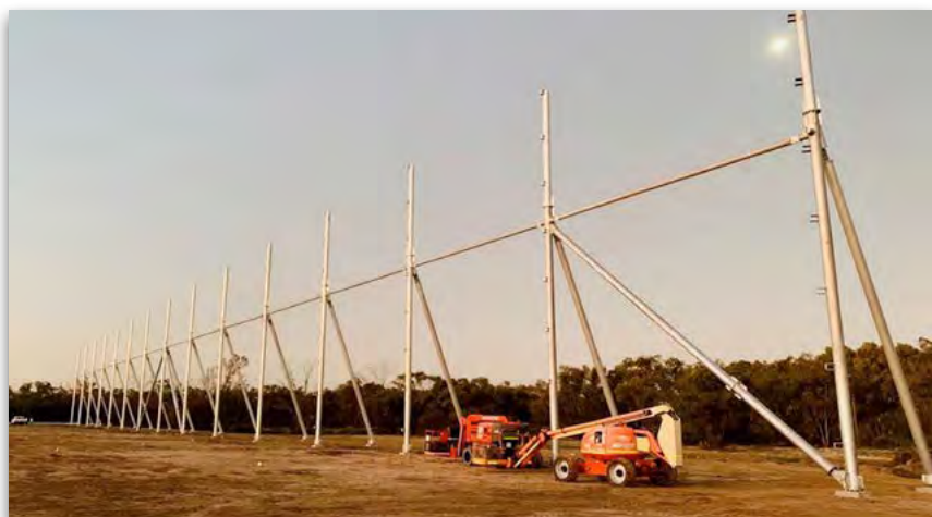
Completion of the back section of the shot curtain supports
