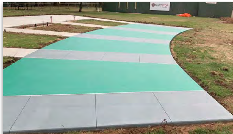
Painting and shaping up of the pads
