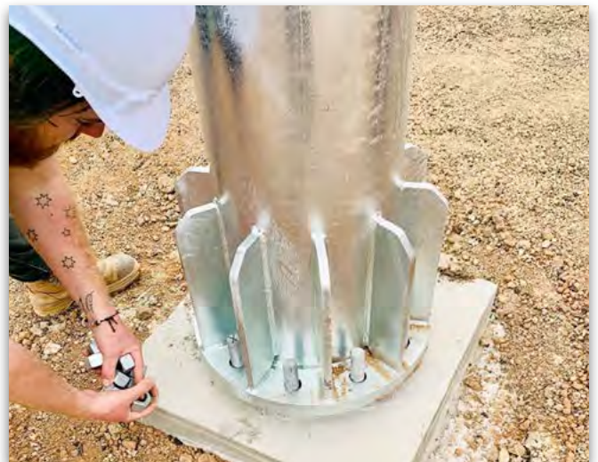
Fixing of support posts to the base
