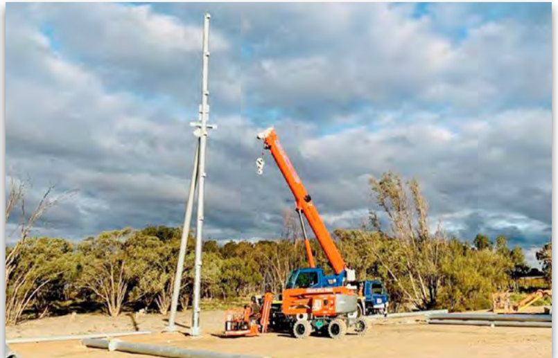
Installation of the first post with the support
