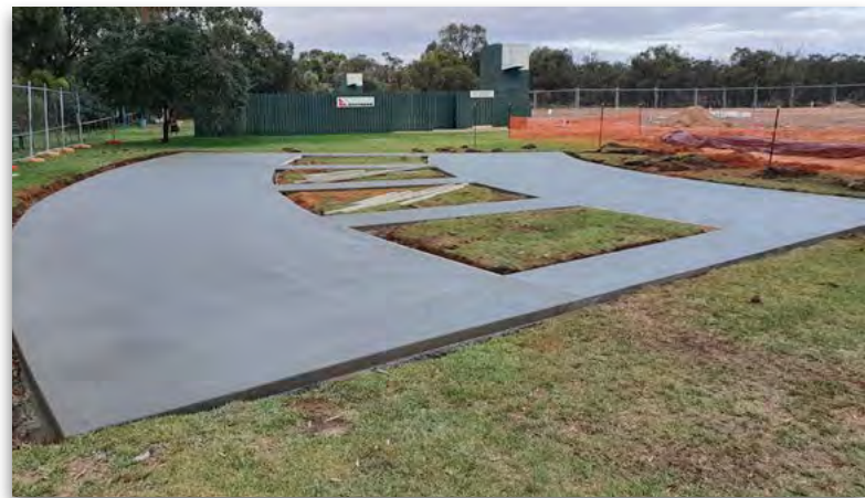
Concrete curing before painting
