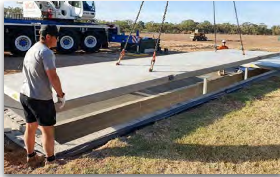
Left: View from the entrance into the Olympic trench Above: Final ceiling piece being placed into position Right: Ceiling installation completed Below: Olympic trench following final fittings and painting
