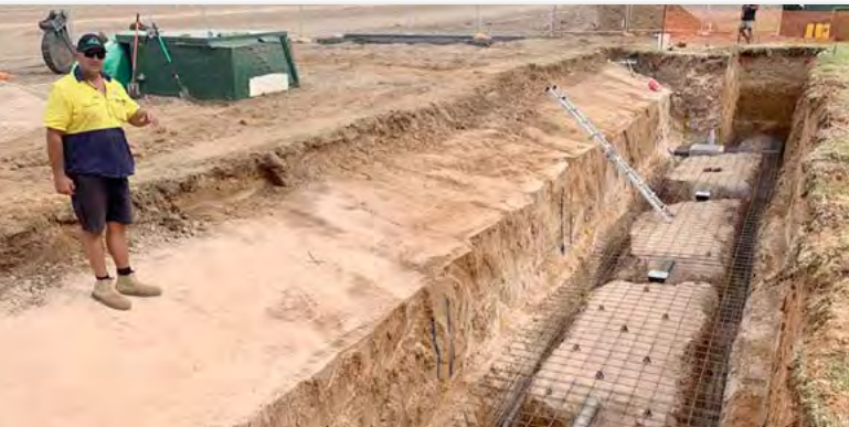
Preparation before pouring of concrete floor
