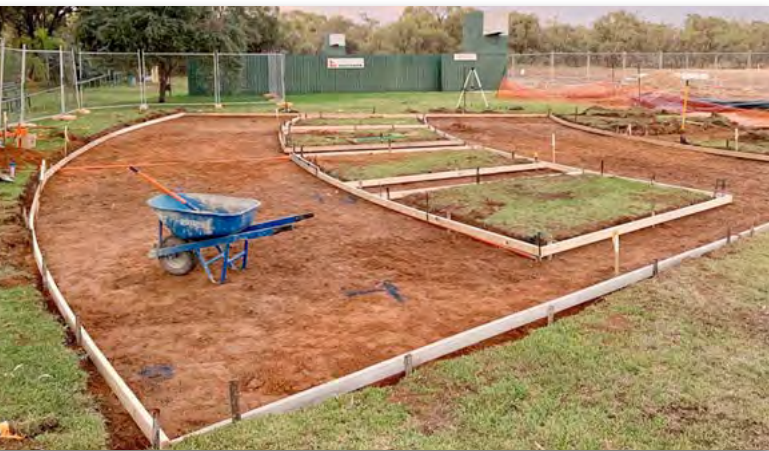
Preparation prior to the laying of reinforcement and concrete
