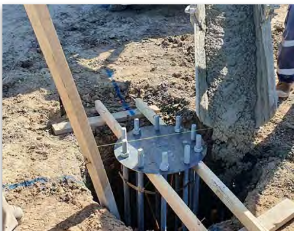
Pouring of concrete to fix the supporting pads
