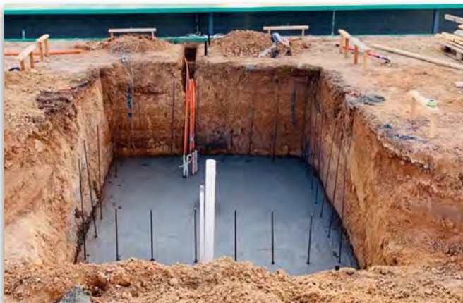
Concrete flooring for trap 2
