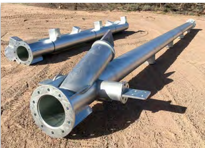
Delivery of curtain post. The 2 pieces go together to provide one post
