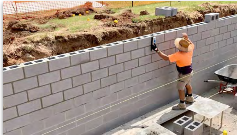
The walls are reinforced with rods and concrete
