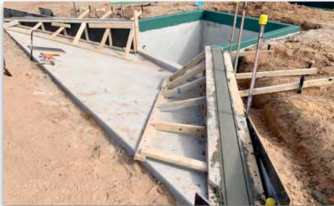
Formwork in concreting to finish off track 2
