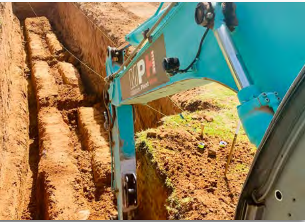
New Olympic trench being dug
