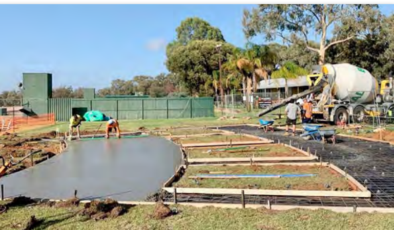
Pouring and levelling of concrete
