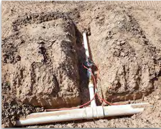
Irrigation system installed for the planting of grass
