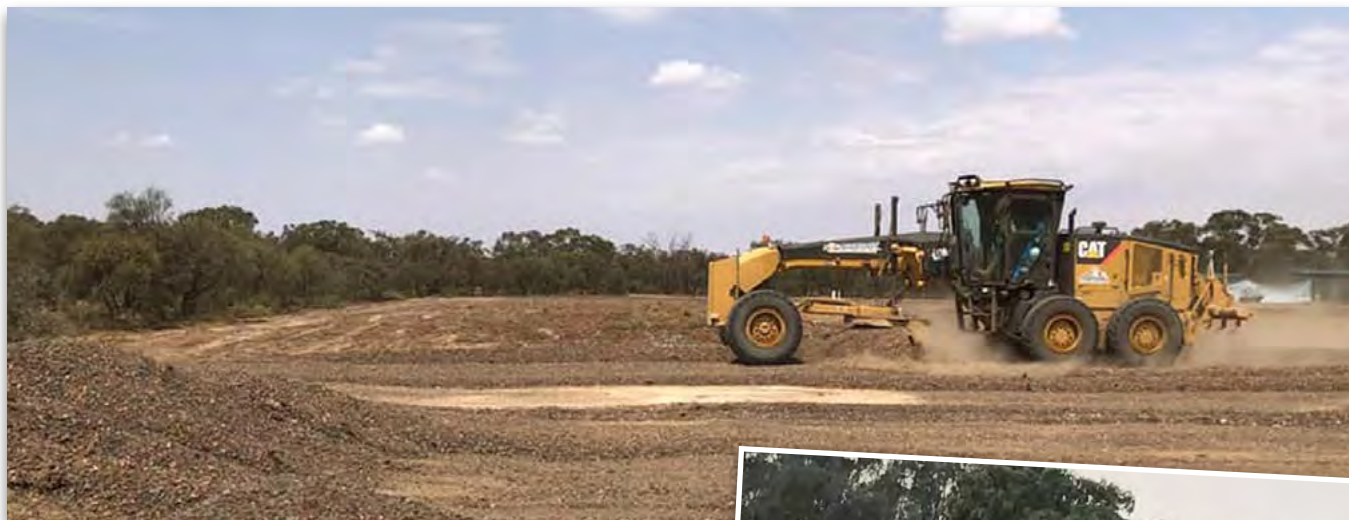
Above: All projects commenced with the area being cleared
