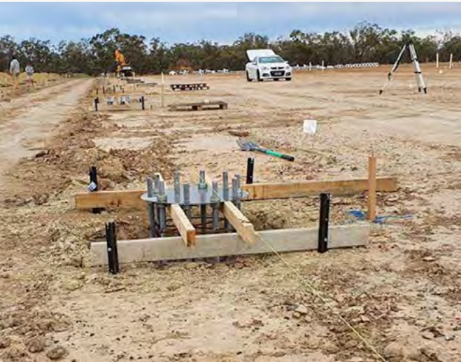
Preparation of foundation pads for the shot curtain
