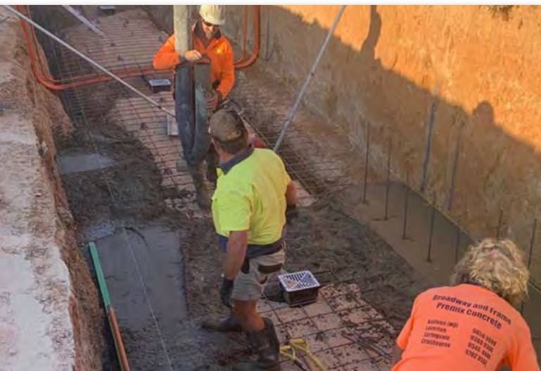
Above: Concrete floor being poured
