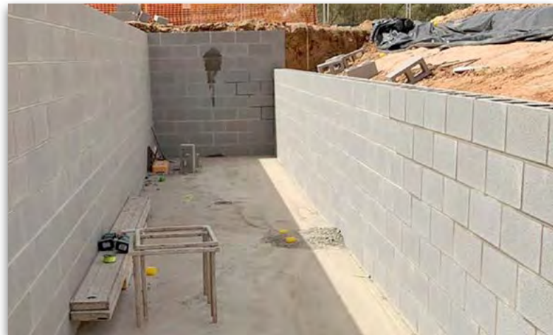
Above: Completed trench prior to the installation of the ceiling
