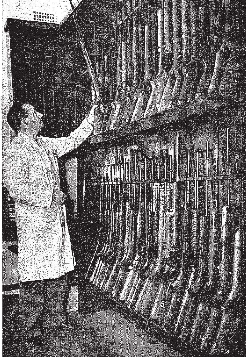
Some of the 170 rifles and shotguns used to test ammunition at the proofing range of the Deer Park Ammunition Factory.
