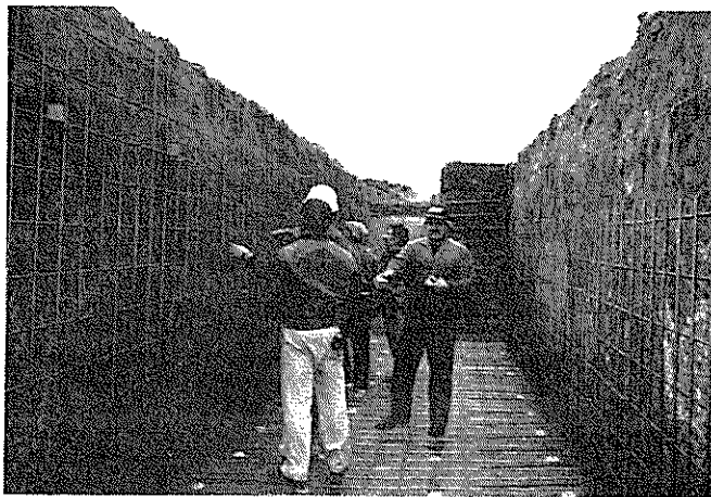
• Setting up the re-enforcing material for the first Trench layout.
