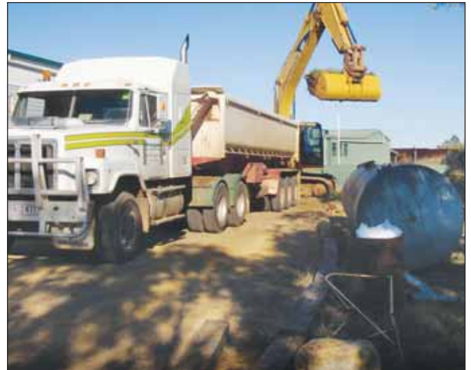
Hoisting septic tank into position
