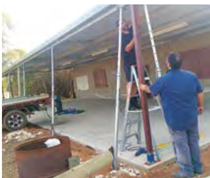
New concreted verandah area
